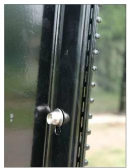
Finally secure the upper 4 bolts incl. cap & cover plate on middle and end post
