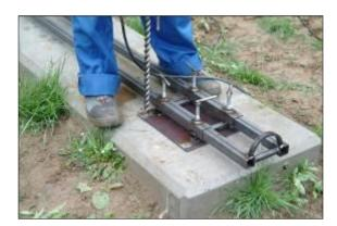
Predrill holes for the base plate
