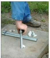
Press the treaded rods by turning round!! Pre-adjust the bar with a nut at the exact height
