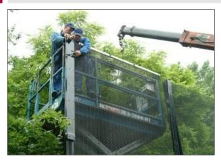
Set up the next panel and fix temporarily to the 2nd and 3th post
