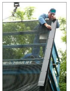
Fix temporarily by means of bolts while holding the panel in position with the crane
