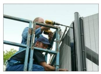
Finally secure the 4 upper bolts at left and right side whilst holding the panel in position with the crane
