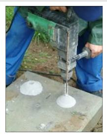
Drill to the size of the predrilled holes
